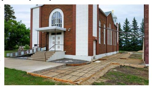
By now the base for pouring the concrete sidewalk, not only adjacent to the leakage site but all along the south wall of the temple, is ready, and is going to be poured very soon. So, if anyone would like to contribute, you are welcome and blessed!
